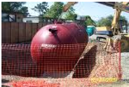
Installation of underground cistern
