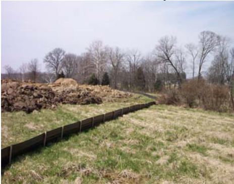
Silt fence protecting exposed soil run-off
