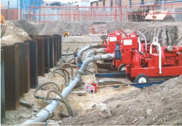
Dewatering of an excavation
