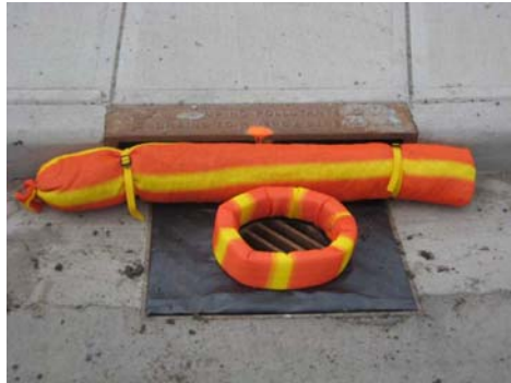
Storm drain sediment protection
