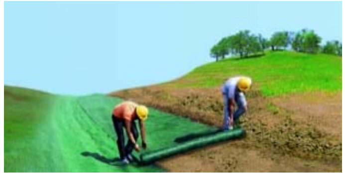
Installation of erosion control blankets
